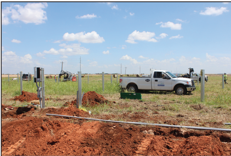
Early construction of SWRE's Frederick solar field
